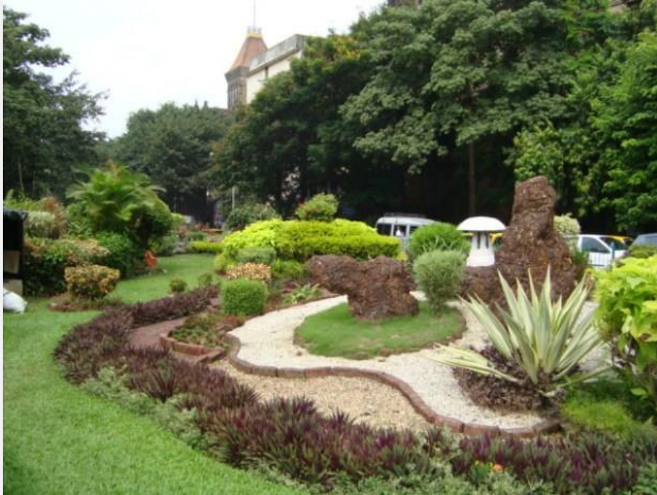
The Orchid in Mumbai has a Sewage Treatment Plant on its roof to treat all waste water
