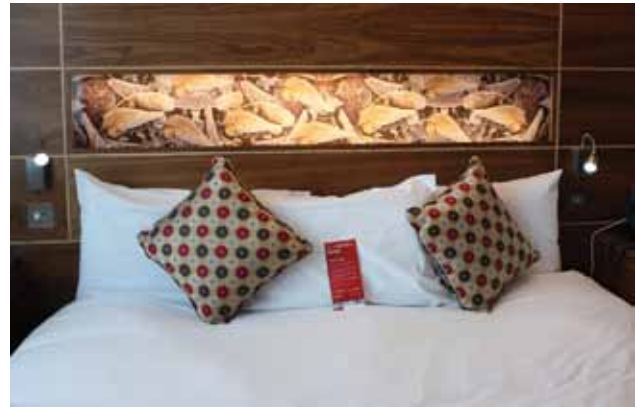
Fig.6 Concealed T8 high efficiency tubular fluorescent and LED reading lights
